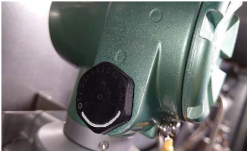
Fig. 5 Ex e blanking element installed to an Ex d equipment
