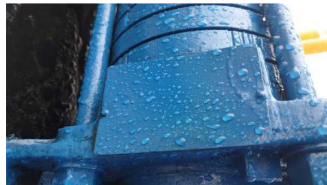
Fig. 2 Ex equipment installed in zone 2 but with its label plate being painted
